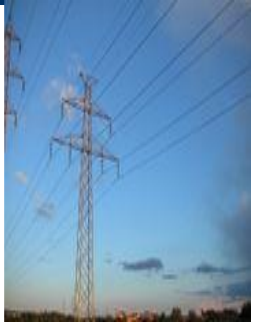
Power lines showing double circuits
