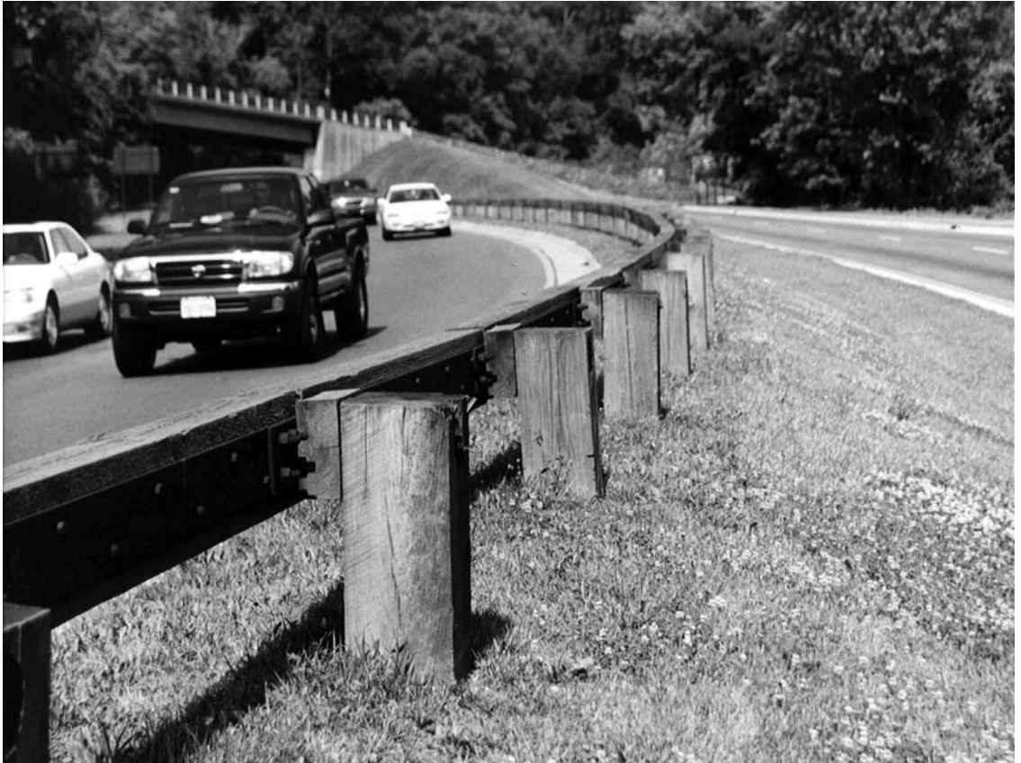
Figure 15.6 Steel-Backed Timber Guardrail
