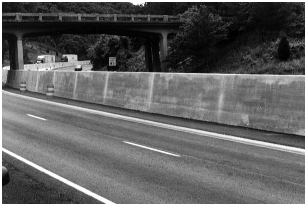
Figure 15.7 Single-Slope Concrete Median Barrier
