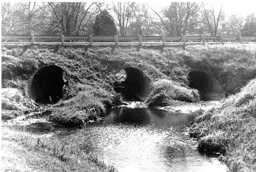
(a) Corrugated metal arch culvert (ARMCO)
