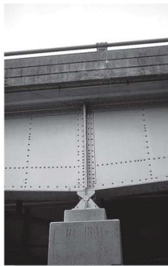
Typical pin used to support the steel girder of a railroad bridge.
